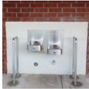
ADA drinking fountains
