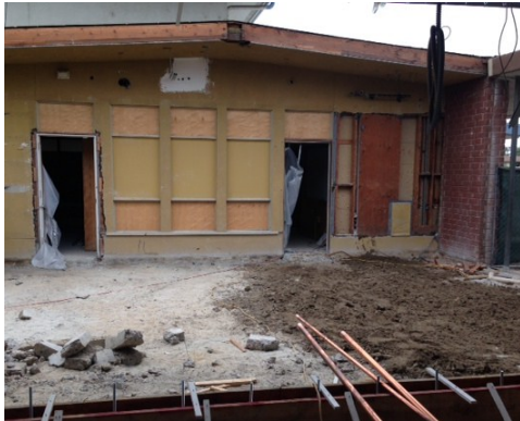
Demolition of Office Workroom
