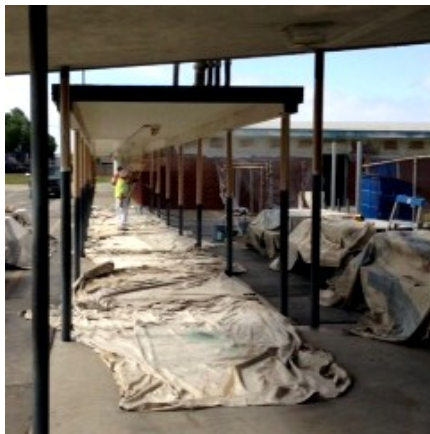
Painting covered walkways
