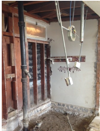
Demolition of staff restrooms
