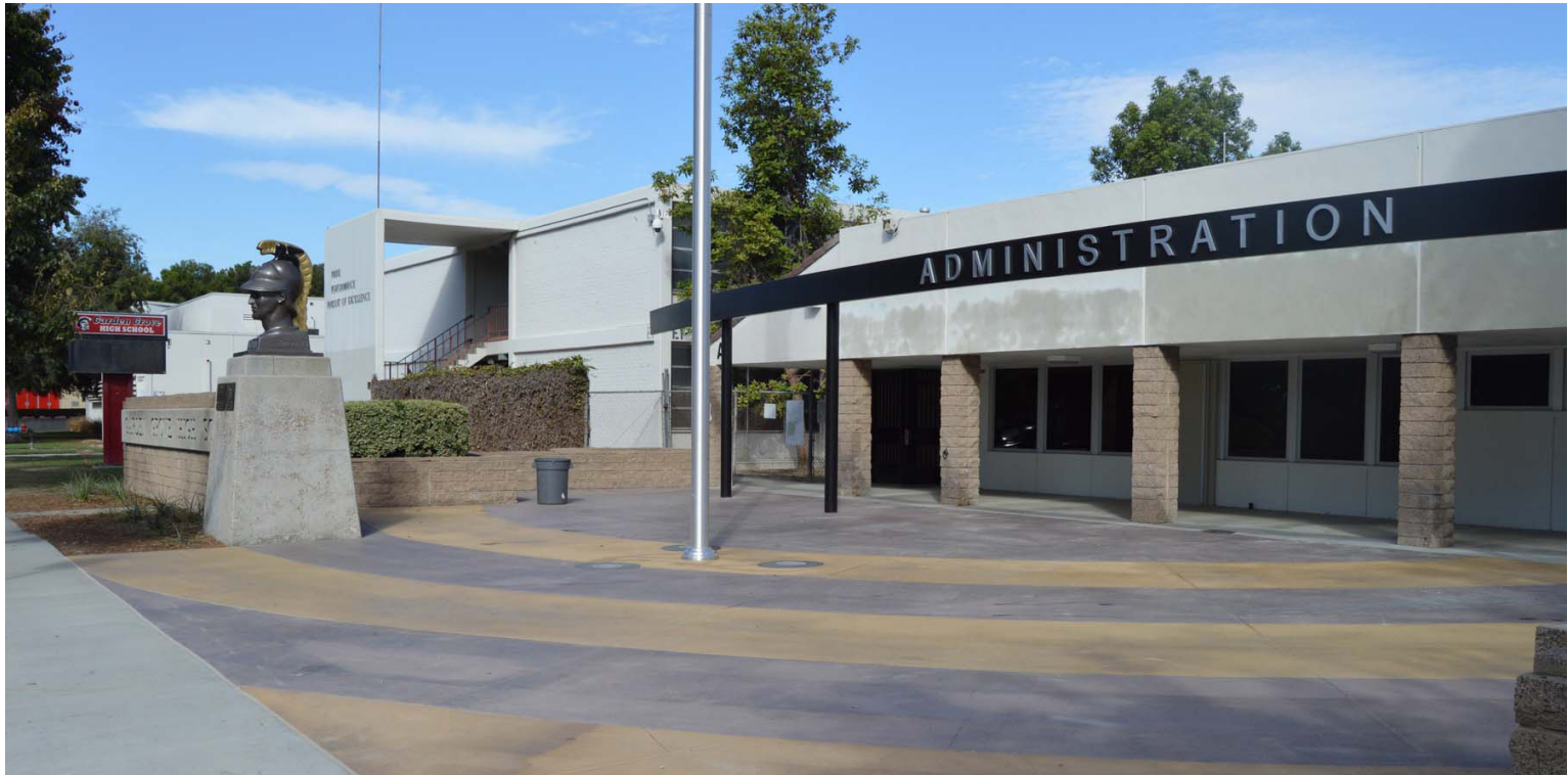
The modernized entrance and front office at Garden Grove High School due to Measure A.
